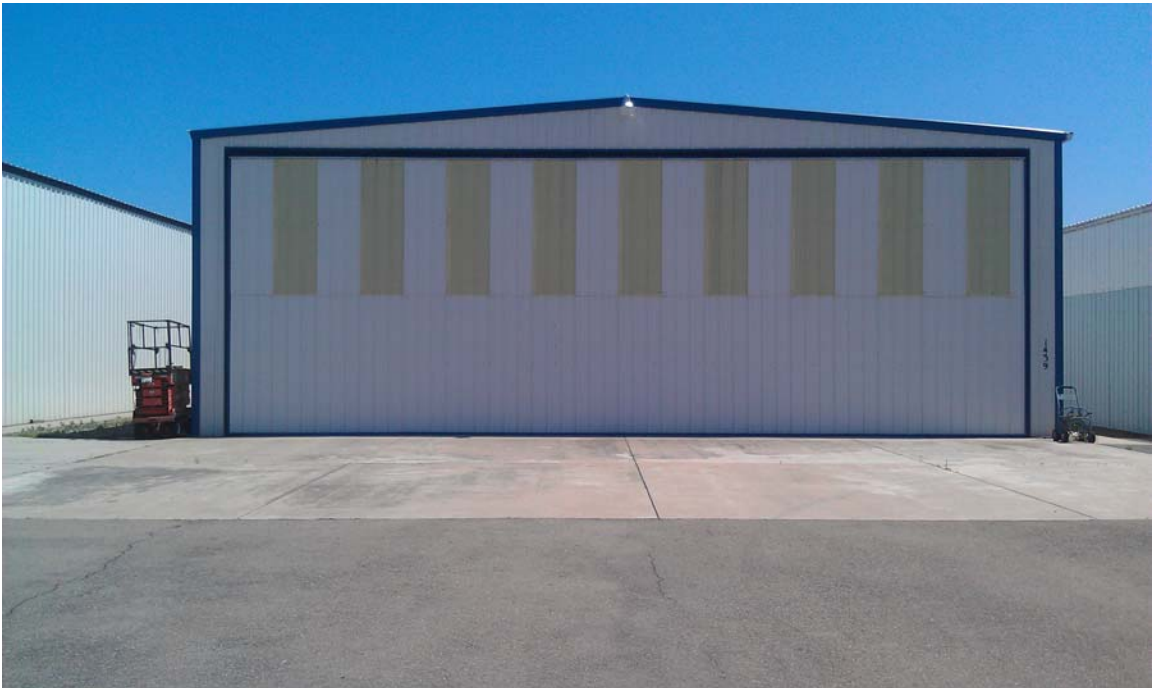
Looking south at Hangar door.
