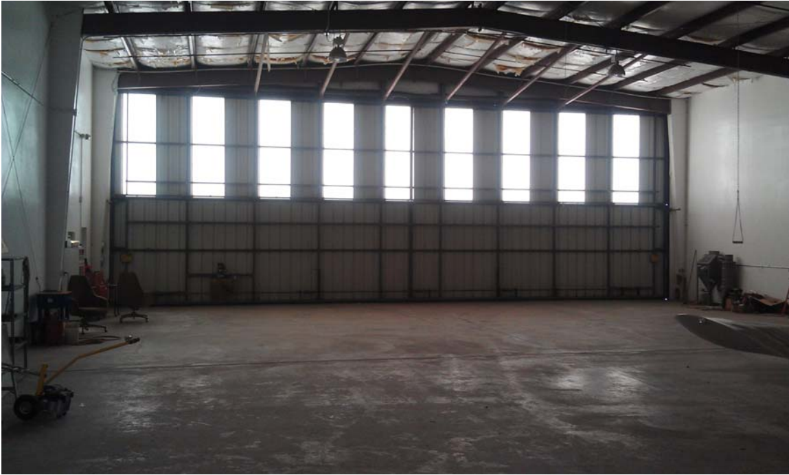
Inside view of Hangar door.
