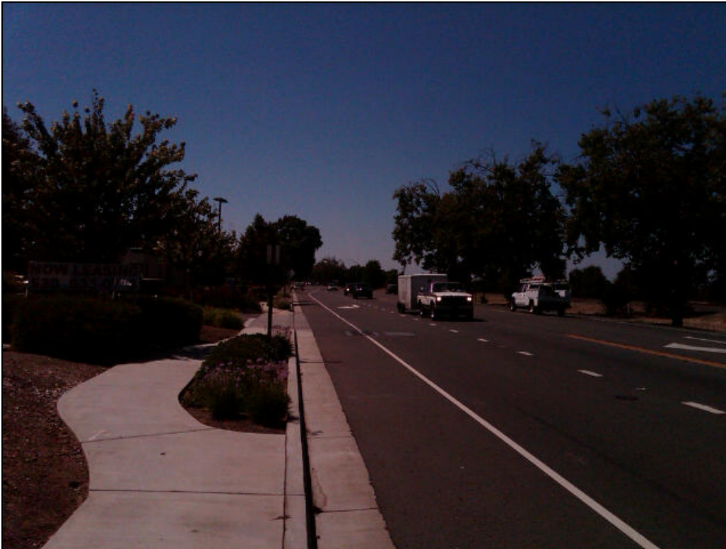
VIEW NORTHBOUND ON HIGHWAY 65
